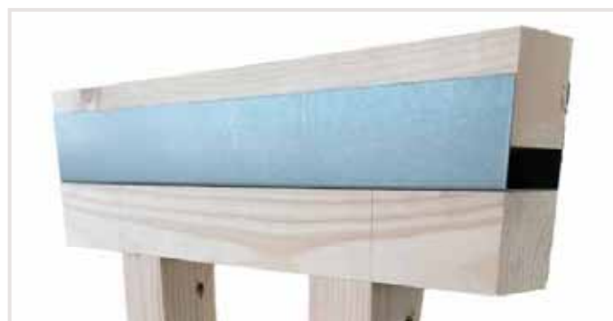
Sliding connection with ClayTec ceiling sliding profile and ceiling transom
