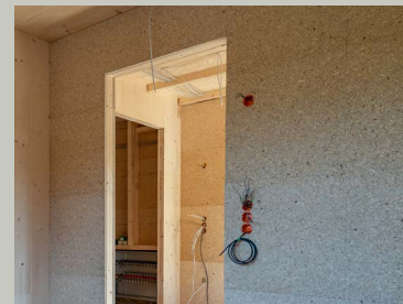
❶ Construction in timber frame design, interior cladding of the walls with esb-Plus wood-based panels.
