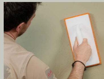
❹ ❺ YOSIMA clay design plaster is usually finely grated. Surface finishing should be carried out with only a small amount of water.
