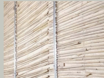
❷ Installation of reed matting St 70 as plaster carrier directly onto the esb-Plus panels.
