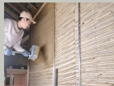
❸ Machine application of ClayTec Clay undercoat plaster with straw
