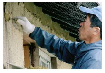
Japan has a centuries-old tradition of clay plasters. The surface design of the clay walls is of prime importance. The best evidence for the cultural significance of this craftsmanship is provided by the multitude of tools with which Japanese plasterers apply, smooth and craft the clay.
