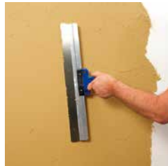
Trowel marks are smoothed out with a finishing spatula
