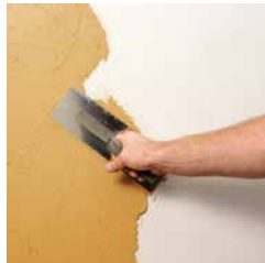
YOSIMA is applied using a trowel.
