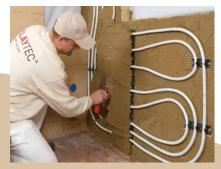
The undercoat plaster is smoothed over the pipe clamp
