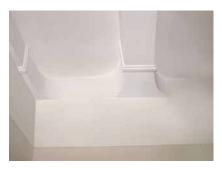
Ceiling with plaster-clad beams, rounded valleys and stucco mouldings
